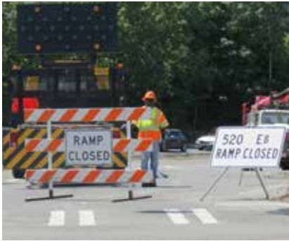
Temporary construction signage for the West Approach Bridge North project.
