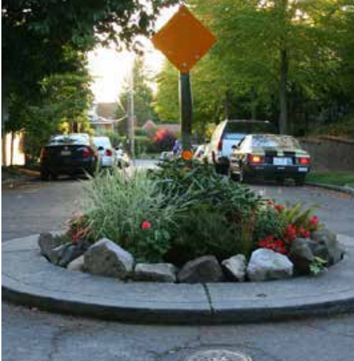
Traffic circles are effective at reducing speeds and the number and severity of collisions at intersections.
