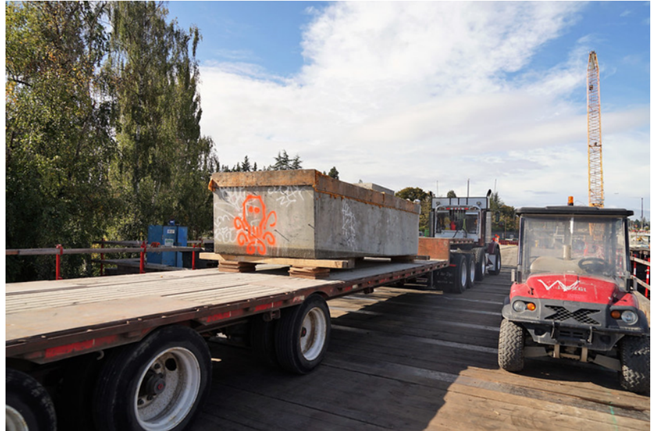
Trucks taking away carefully removed sections of the old SR 520 Bridge
