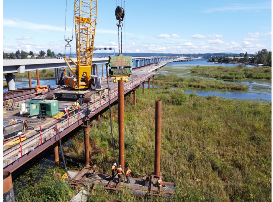
Pile installation in Lake Washington
