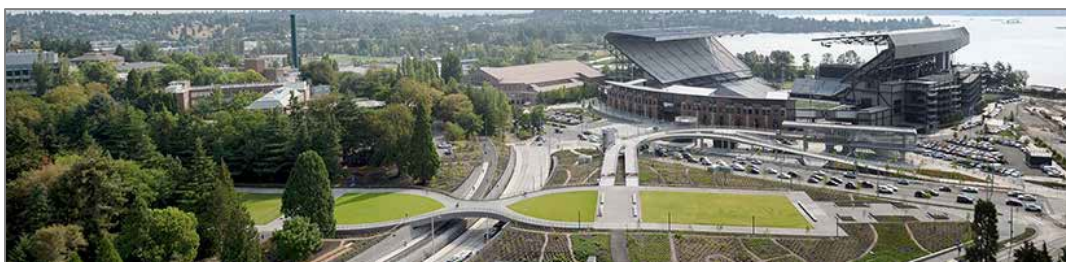
The Montlake Triangle provides a grade-separated crossing over Montlake Boulevard NE for pedestrians and bicyclists.
