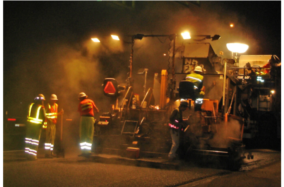
Crews conduct highway paving activities at night
